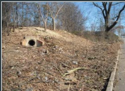
Storm sewers that discharged directly into streets were common in the area due to the lack of a storm drainage collection system.
