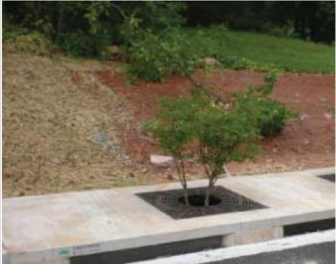
TreePod bioretention filters remove impurities while simultaneously contributing to environmental sustainability.
