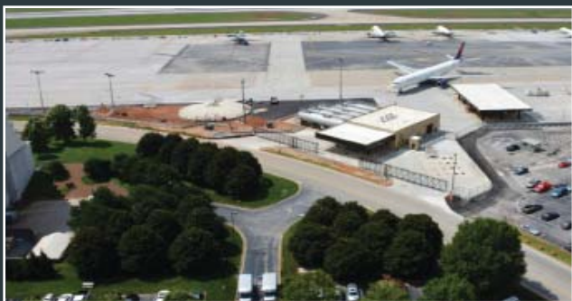
The finished North Airfield Deicing Facility.
