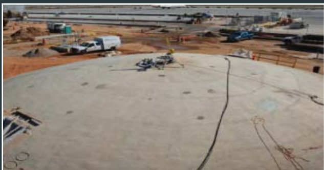
Placing the 2,000,000-gallon+ reclamation tank.
