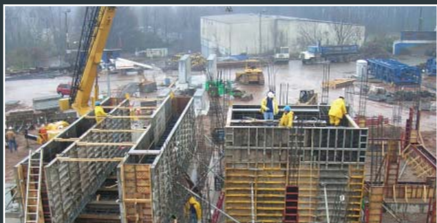
Construction of shredder.
