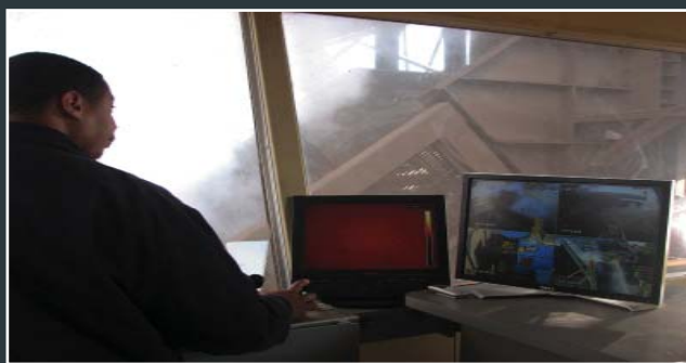
Shredder control room
