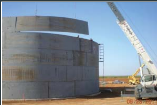
Placing the 2,000,000-gallon+ reclamation tank.
