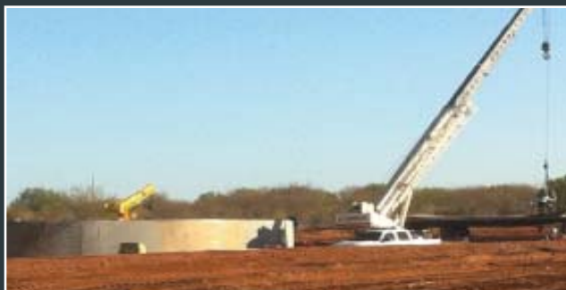
Construction of ringwall.
