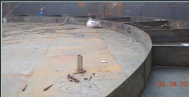
Construction of floating roof.
